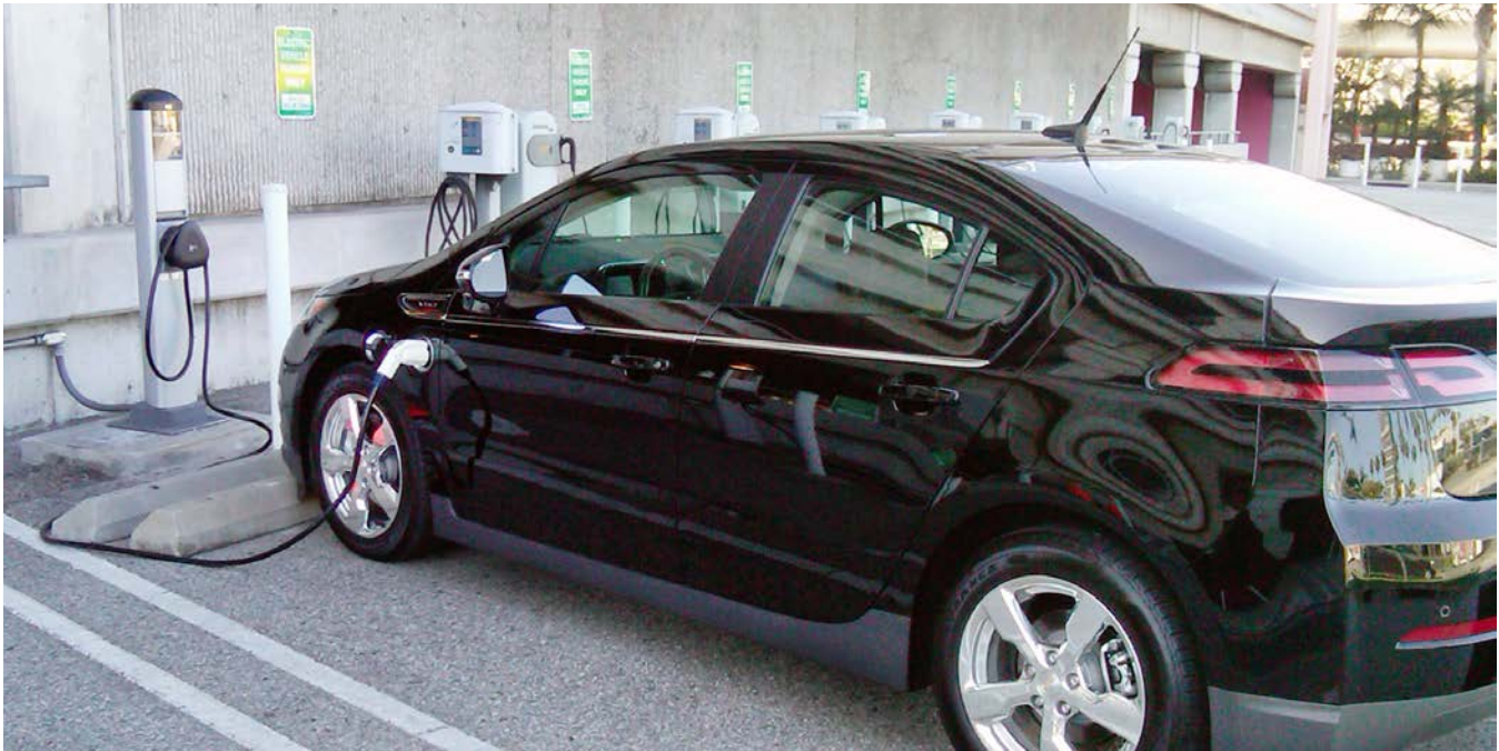
A Chevy Volt charges up with public Level 2 EVSE at Los Angeles International Airport. Photo from Coulomb Technologies
