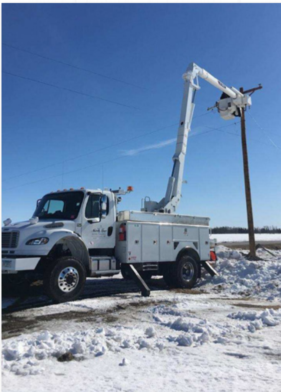
Baudette crew works on Zippel Bay road conversion from single-phase to v-phase.
