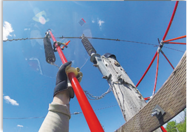
An insulated fiberglass hot stick is used to safely install blink outage mitigation equipment on energized lines.
