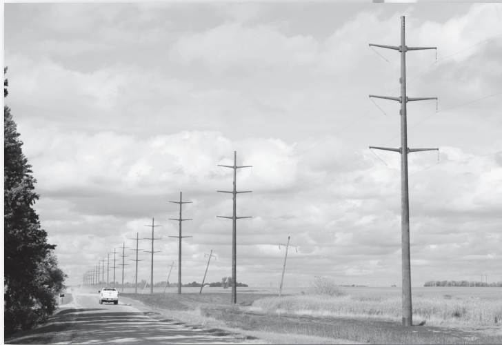
A new 230-kV generator outlet line was constructed between the existing Maple River substation near Fargo, N.D., and the new Pillsbury Wind substation near the wind farm. The line is capable of transmitting 350 MW of wind power.
