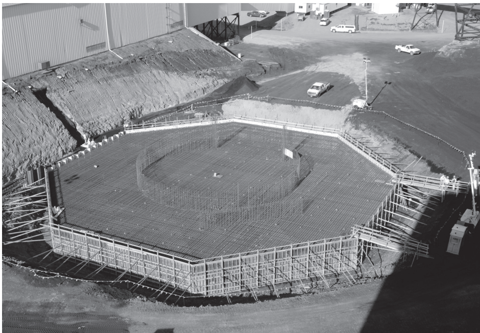
More than 6,000 cubic yards of concrete was required for the base of the new Young 2 stack. Here, the forms and rebar are in place prior to the pour.
