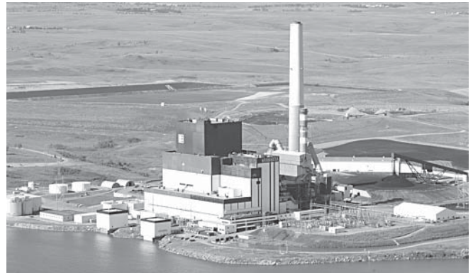
Minnkota is studying the feasibility of a third lignite-fueled generating unit that could be located at the Young Station site near Center, N.D.
